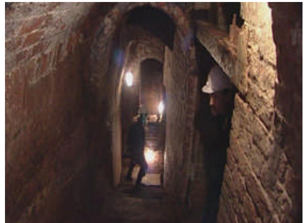
Williamson's tunnels beneath Liverpool
