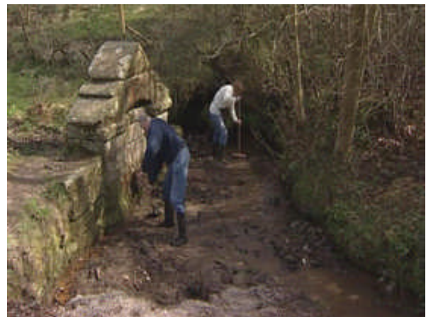
Local volunteers maintaining Ladydale Well
